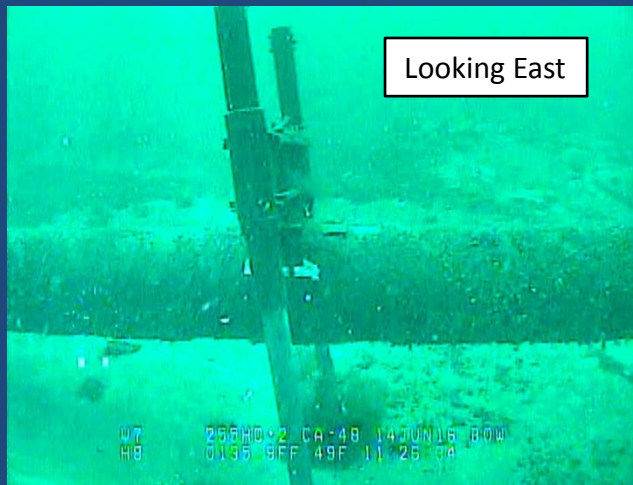
Laterally Deflected Anchor from 2016 Inspection
