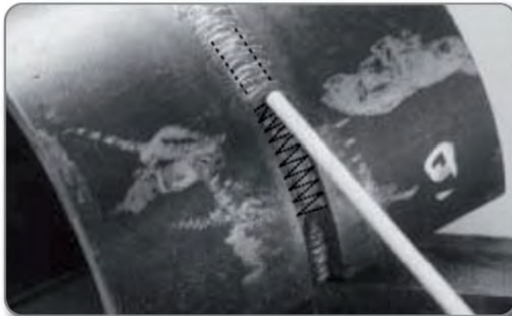
Pipeline Girth Weld Showing Completed Root Pass and Details of Second Pass
