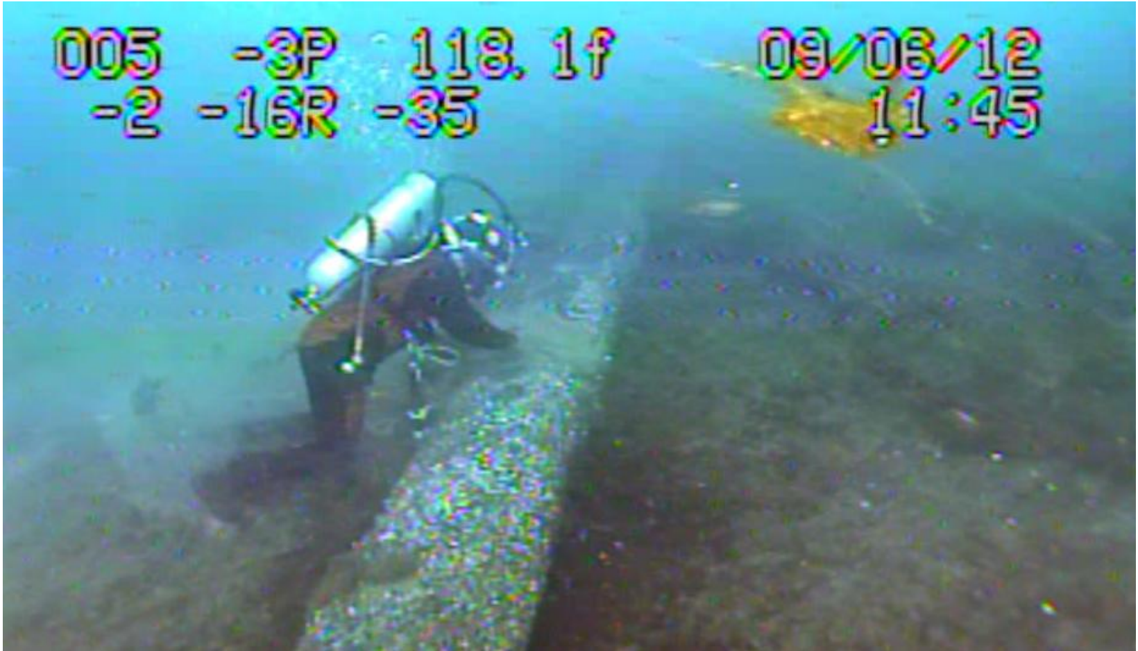
Unsupported Section of Line 5
