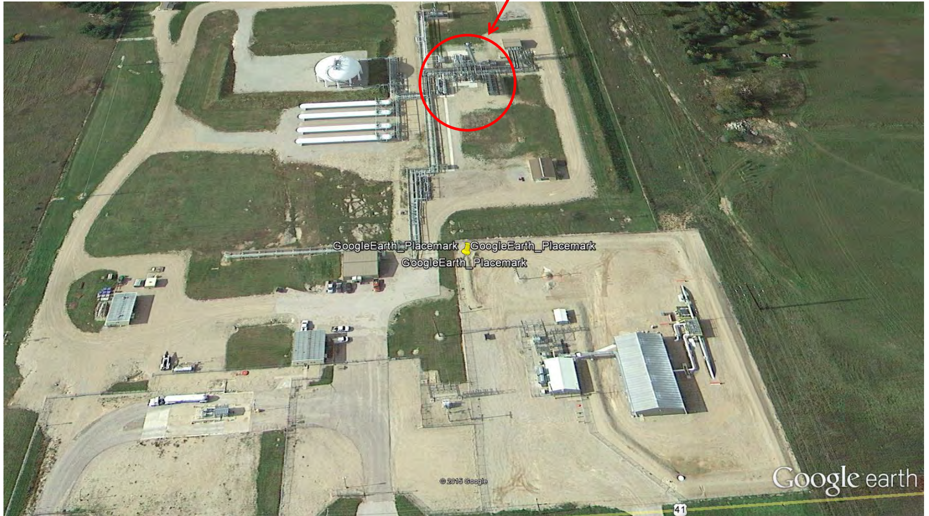
Enbridge -- Rapid River (MI) Propane Facility
