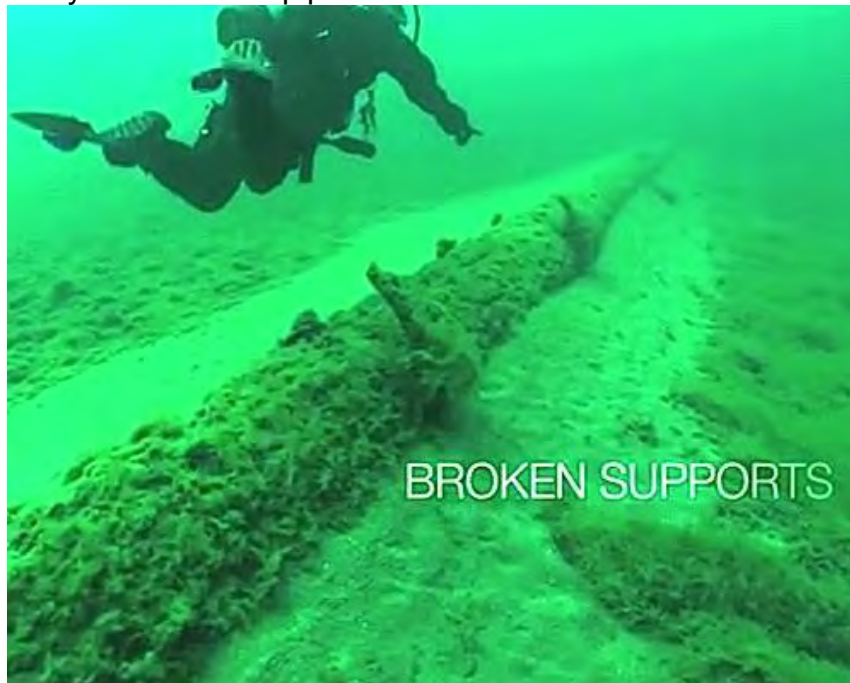
Figure 1. Picture of Line 5 Taken by NWF that Erroneously Identifies Corroded Circumferential Bands as Broken Supports
