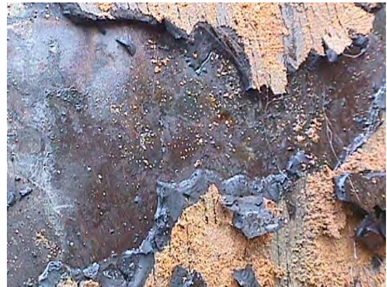
Failed Coal Tar Coating
