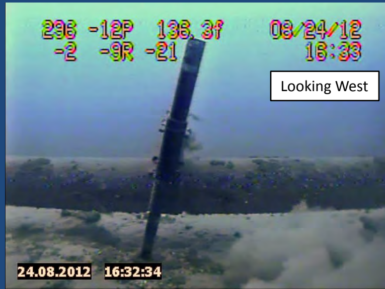
Laterally Deflected Anchor from 2012 Inspection
