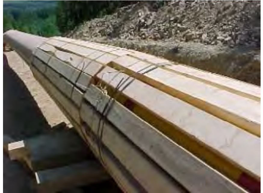
Temporary Lagging on a Pipeline for Abrasion Protection
