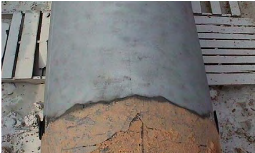
Coal Tar Adhesion Failure
