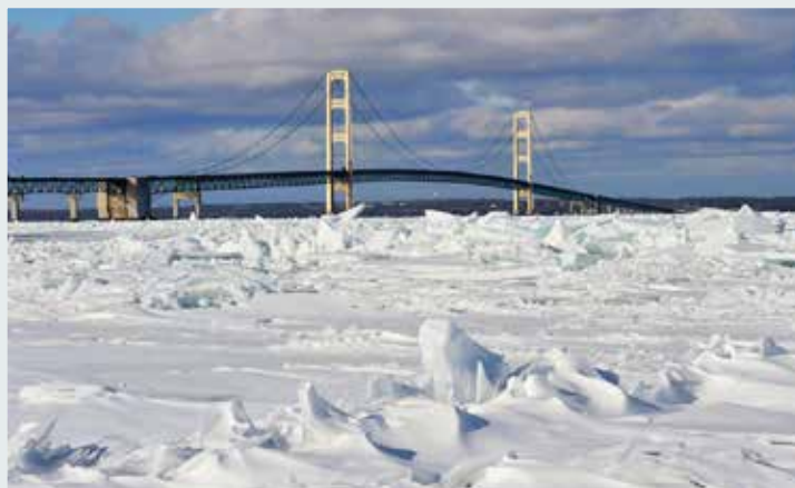
Mackinac Bridge in winter
